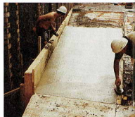
Concrete is poured around the outside of the shutter left and then once it's set, the shutter's collapsed to leave a hole. For the shutter on the right, concrete is poured between the shutters and again, once set, the wooden construction is removed
