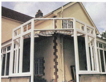
(Above) Pre-cut rafters in position and ready for fixing. The finial is an essential feature as it gives support (Right) This conservatory consists of two spans of tiled roof intersecting at a glazed section. It will create considerable insulation for the main building and will have a sun-trapping corner with the additional advantage of a shaded area. In the summer some conservatories get very hot and blinds may well be required
