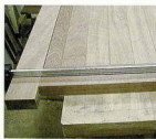
14 Assemble each door using sash cramps across the rails. Check for square by measuring across the diagonals
