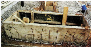
Concrete is poured around the outside of the shutter left and then once it's set, the shutter's collapsed to leave a hole. For the shutter on the right, concrete is poured between the shutters and again, once set, the wooden construction is removed
