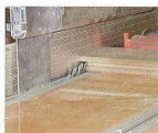
11 Once the shoulders have been cut on the ends of the matchboard, the waste can be sawn away
