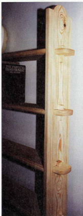
Removable wedges allow for easy dismantling
