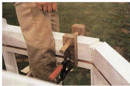
(Left) Making finishing touches to the final – in this case a decorative feature that's also a structural key to the roof
