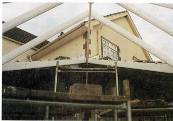
All the main components are all mortice and tenon jointed. (Top) Stub tenons on the transom rail sections with step shoulders to accommodate the rebate lines (Right) A through mortice used for extra strength, with step shoulders again to accommodate the rebate lines
